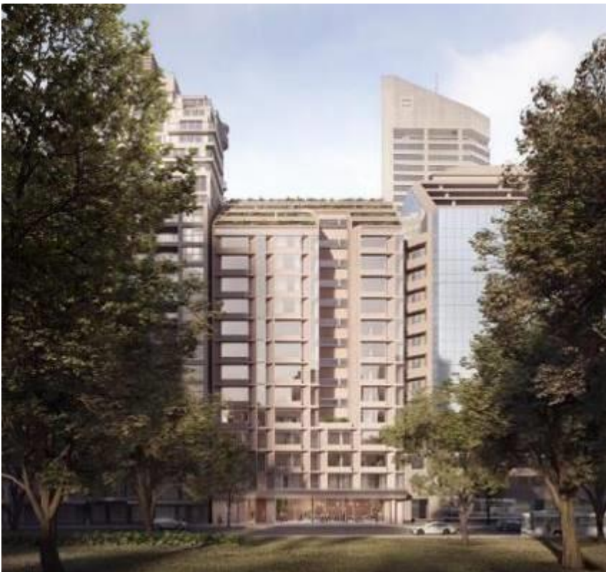
Figure 21: Proposed photomontage of the Elizabeth St elevation, view from Hyde Park facing west
