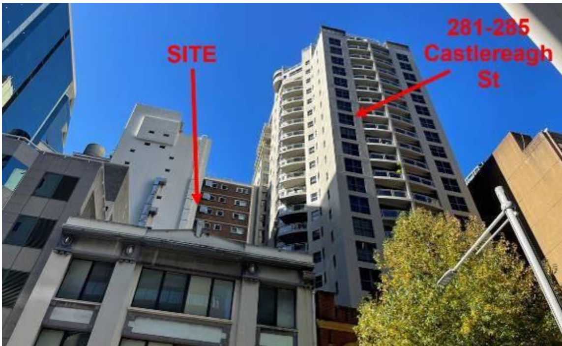
Figure 9: Upward view of site and adjoining residential development to the south
