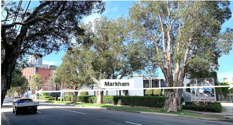
Figure 43: Frontage of the Markham commercial development site at 22 O'Riordan Street.
