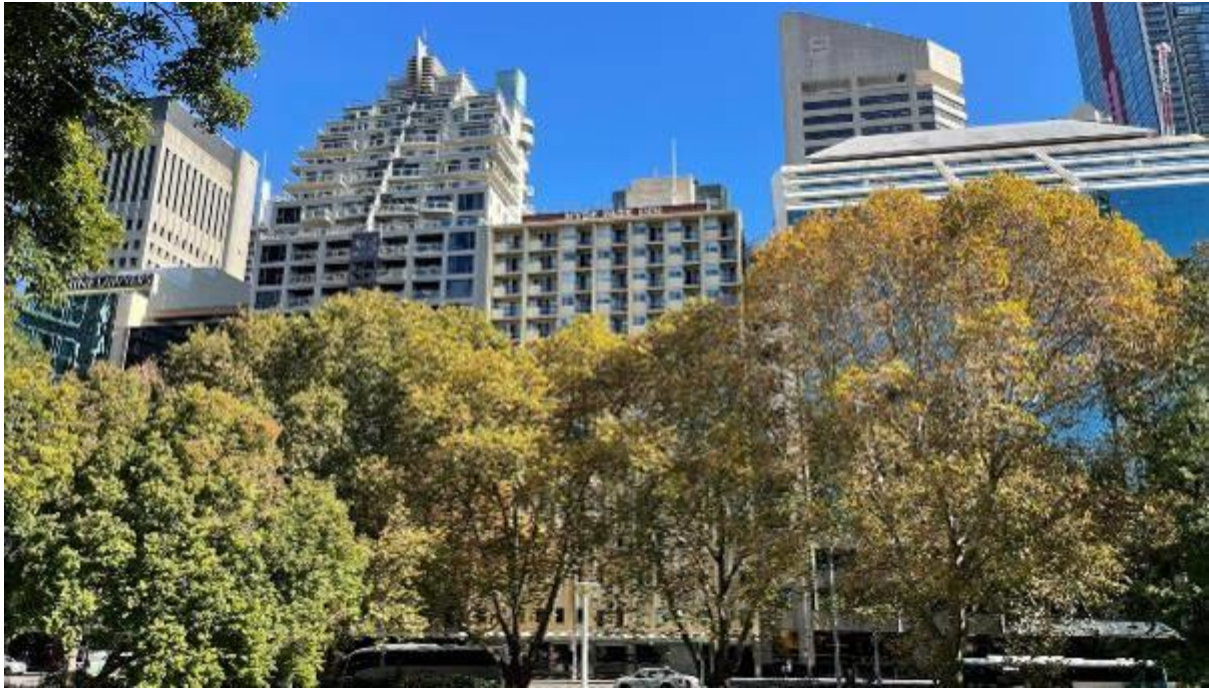
Figure 4: Site's frontage to Elizabeth Street, view from Hyde Park facing west
