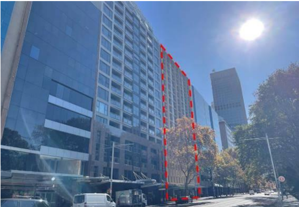
Figure 7: Site and adjoining buildings along Elizabeth Street, facing north
