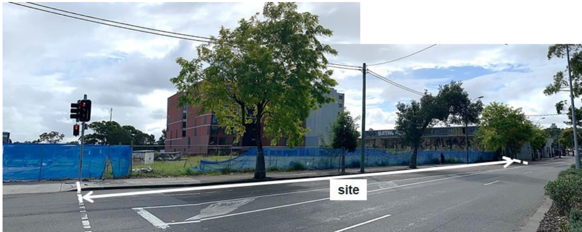
Figure 6: Botany Road frontage of subject site.
