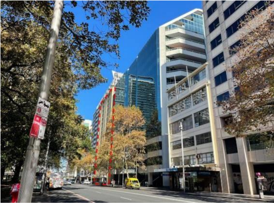
Figure 6: Site and adjoining buildings along Elizabeth Street, facing south
