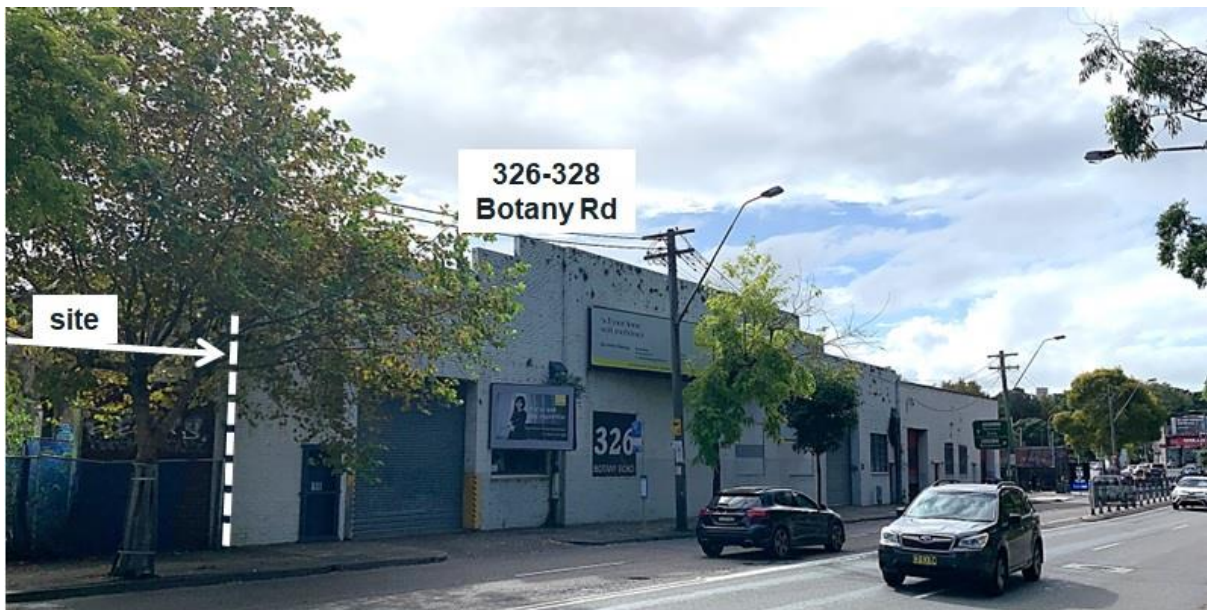
Figure 9: Property at 326-328 Botany Road adjacent to the north of the subject site.
