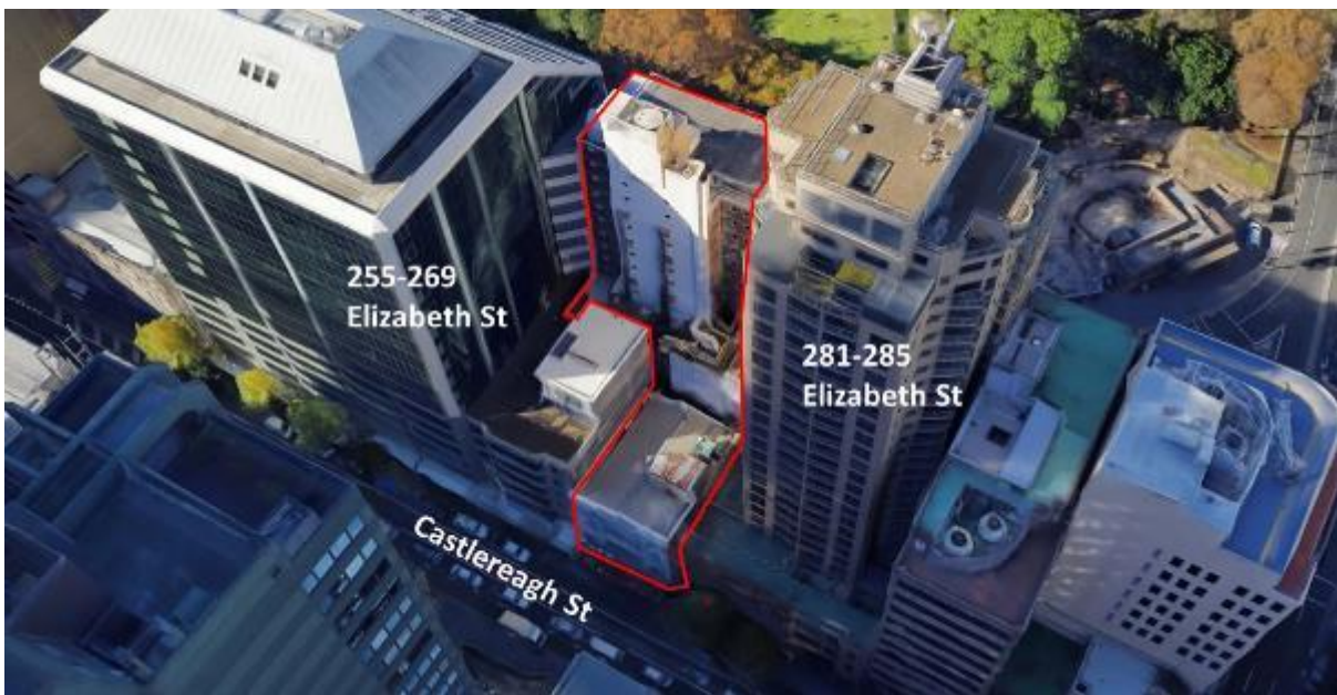
Figure 3: Aerial view of 262-266 Castlereagh Street and adjoining properties
