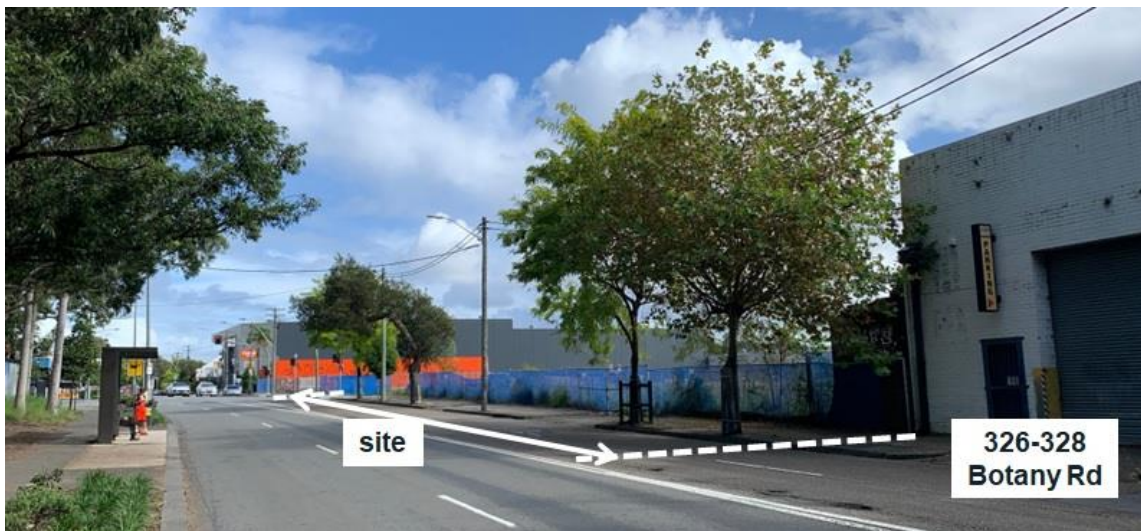
Figure 7: Botany Road frontage of subject site, looking south along Botany Road.
