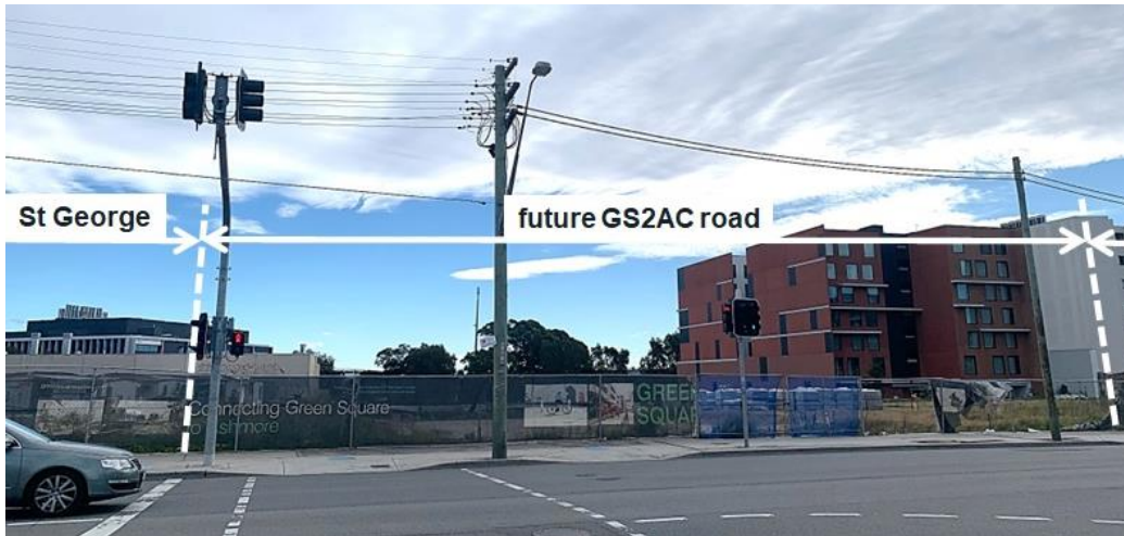
Figure 3: Botany Road frontage of future GS2AC Road.
